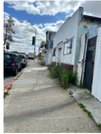
Figure 5. Unkept sidewalk between 63rd St. & 65th St. along Imperial Ave.
