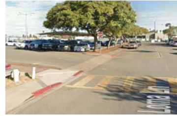
Figure 4. The exit of school parking lot needs a clear "Do Not Enter" sign and the crosswalk on Loma Ln. needs a pedestrian crossing road sign.
