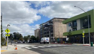
Figure 1. Well maintained sidewalk with flashing light crosswalk on Hartley St. & 47th St.
