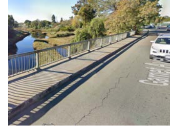
Figure 6. Narrow sidewalk on Rose Creek bridge
