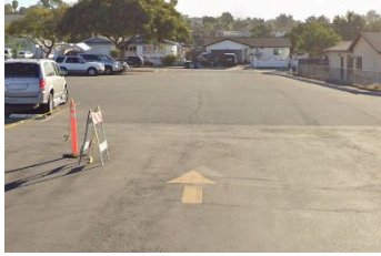
Figure 3. Traffic direction arrows are missing on one half of the school parking lot.
