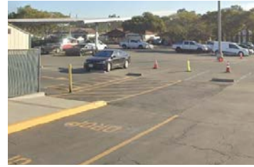
Figure 2. The walkway that leads into the school parking lot needs to be extended for families to safely cross traffic.
