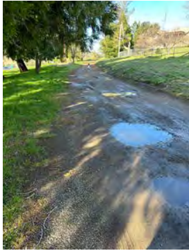
Figure 3. Mud and puddles on the dirt path on the way to school on Cape Horn Ave.
