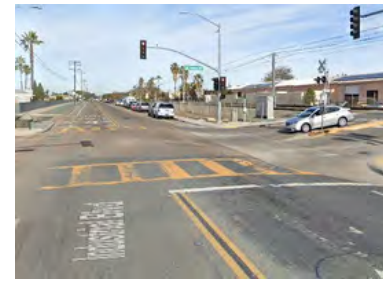
Figure 6. Faded crosswalks on the corner of Industrial Blvd. & Naples St.
