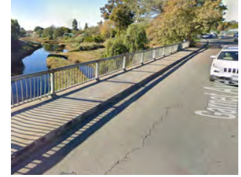
Figure 6. Narrow sidewalk on Rose Creek bridge
