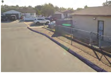
Figure 1. Dirt path that leads to Loma Verde Elementary from Loma Ln. needs pavement and maintenance.
