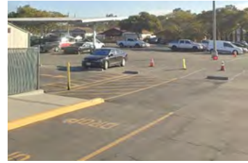
Figure 2. The walkway that leads into the school parking lot needs to be extended for families to safely cross traffic.
