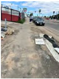
Figure 6. Unkept sidewalk near the intersection of 65th St. & Imperial Ave.
