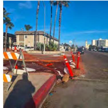
Figure 5. Construction blocking sidewalk at the corner of Orange Ave. & Central Ave.
