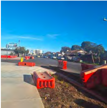
Figure 4. Construction barriers knocked down at the corner of Orange Ave. & 39th St.
