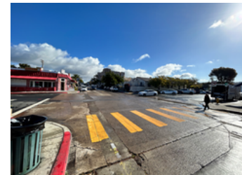
4-stop intersection between Newton Ave and Beardsley St lacks labeled crosswalks
