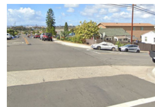
Unlabeled crosswalks at the intersection of S 40th St & Gamma St
